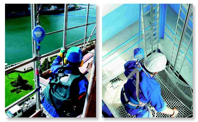
Brake values, which you can see on the brake diagram opposite, are independent of any weather situation or application and far below the 6 KN limit specified by the DIN EN standard.
